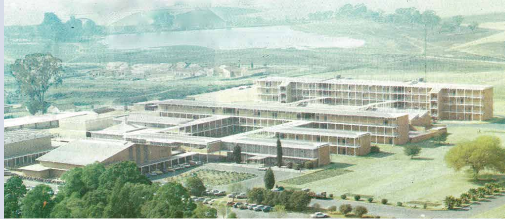
Aerial view of the College
