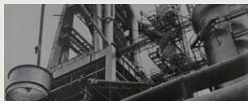
Iscor blast furnace D
