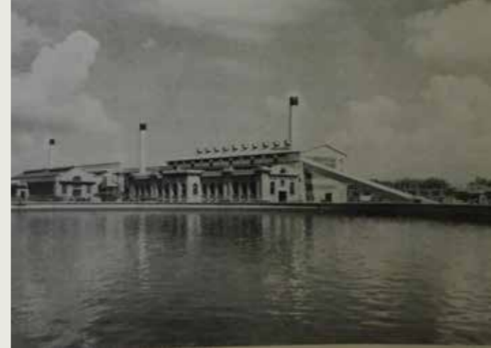
The pumping station at Vereeniging
