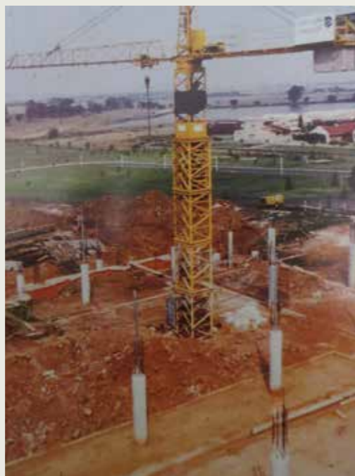
Construction begins on land donated by Vesco to the College – 1964
