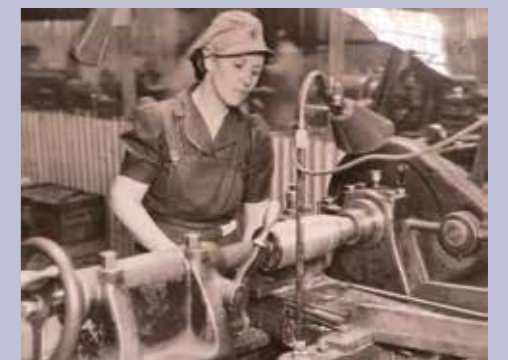
Machining of outer cannon shells during World War II at the Vanderbijlpark Works
