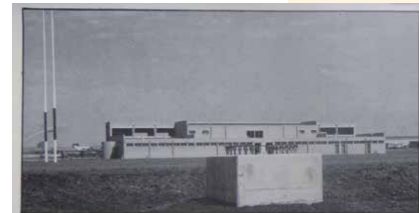
The lighting on some of the fields at the Isak Steyl Stadium will be of provincial colour TV standard. In front is a basis of one of the masts for these floodlights.
