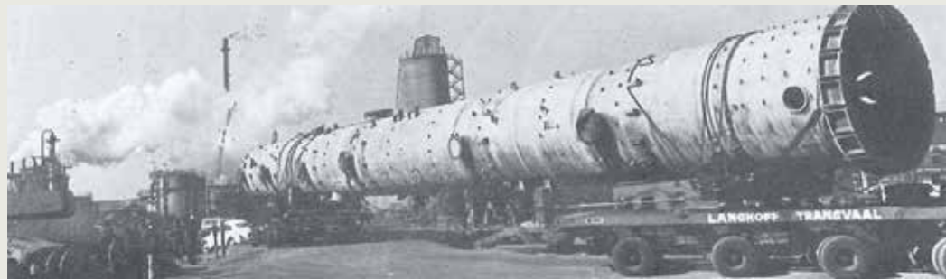
Rectisol Tower for Sasol
